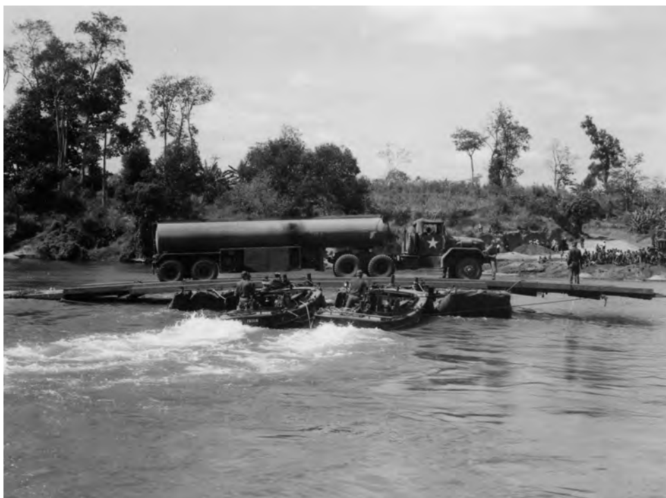
An M4T6 raft carries a 20th Engineer Battalion vehicle across the Ea Krong River on the way to build a new C-130 airstrip at Duc Lap Special Forces camp.
